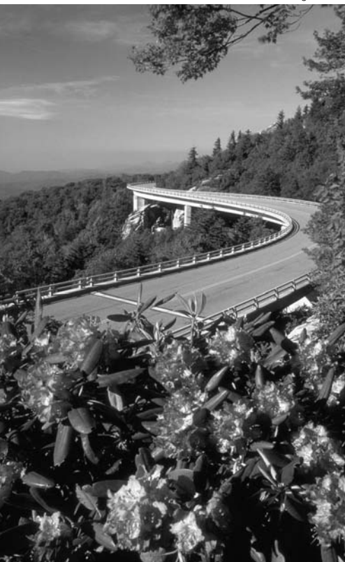
The Linn Cove Viaduct on the Blue Ridge Parkway
